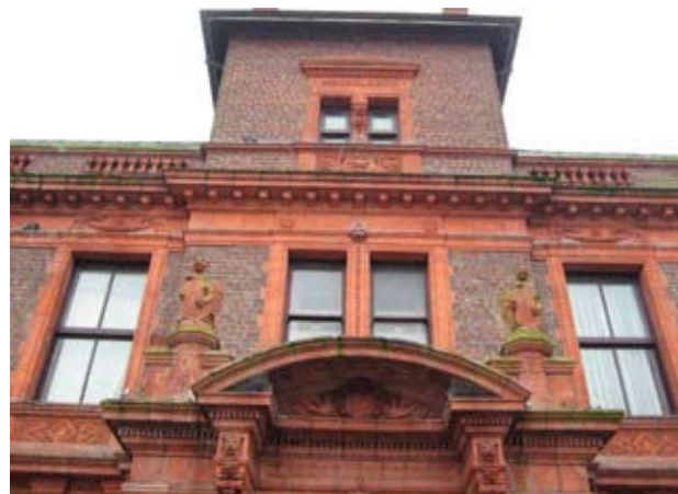
The old Town Hall, built 1885, is being converted to a hotel The old Widnes Town Hall is a magnificent centre-piece to the square, but has been under-used for many years. Its proposed conversion to a 'Boutique Hotel' will bring fresh life. The square itself lacks activity, enclosure or shelter, and needs further thought.
